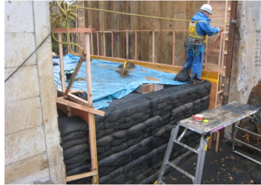
Figure 4. Wall face of the approach block of cement-mixed gravelly soil under construction (27 November 2008)
